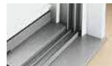
An extended insect screen track is required for two-panel active-passive or passive-active hinged doors that use gliding insect screens.
