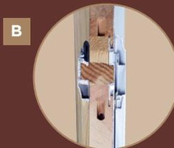
**B** Locking flush bolts at the head and sill for increased structural performance and security
