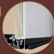
**B** Durable stainless steel track on interior of the sill for smooth sliding operation
