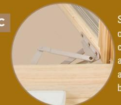
**C** Smooth-functioning operating hardware, concealed for a clean appearance and allowing sash to open beyond a full 90°
