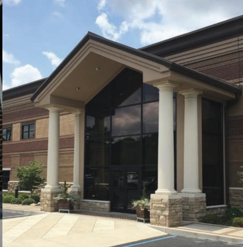
Lightweight fiberglass columns that are large in size and easy to install.
