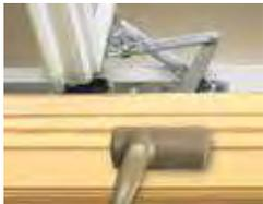
Corrosion-resistant hinge and operator arm hardware on casement, awning and venting transom windows is designed for applications in harsh and corrosive environments such as heavy industrial or coastal areas.\*\* Shown on a 400 Series casement window.
