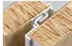
A full-length combination weatherstrip/interlock system provides a flexible seal at the meeting stile. Shown above on a 400 Series Frenchwood® gliding patio door.
