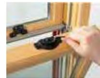
Traditional spoon lock design has an integrated tilt-to-clean feature, so both sash can be cleaned from the inside.
